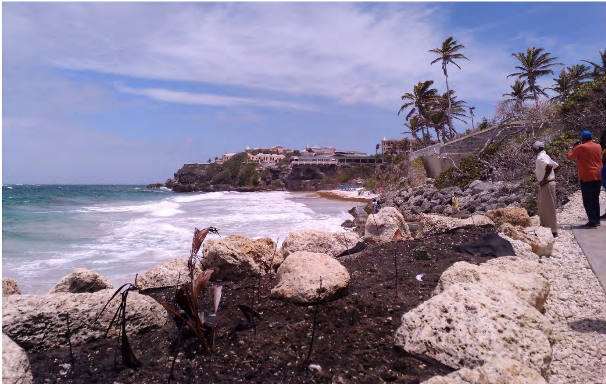
Figure D.2. Ad-hoc coastal protection schemes at Crane Beach
